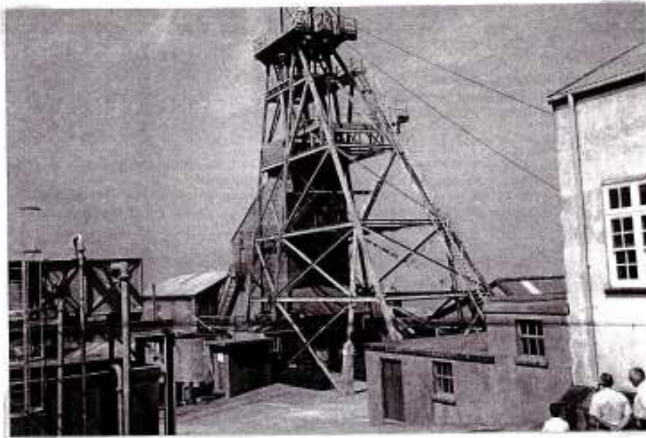
This is the main shaft of Geevor Mine , now closed
